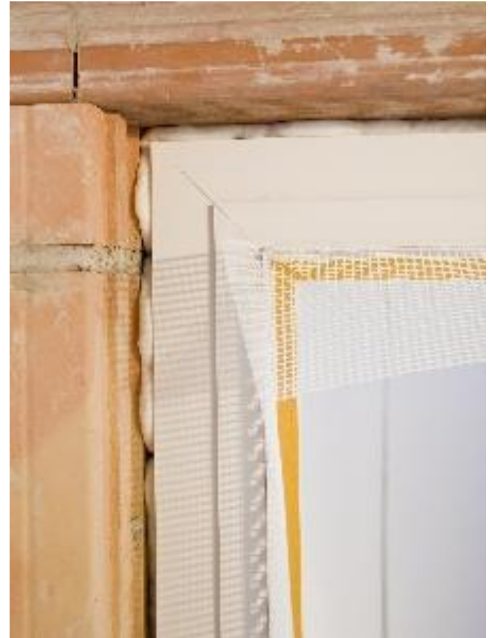
Window frames without wooden frame
